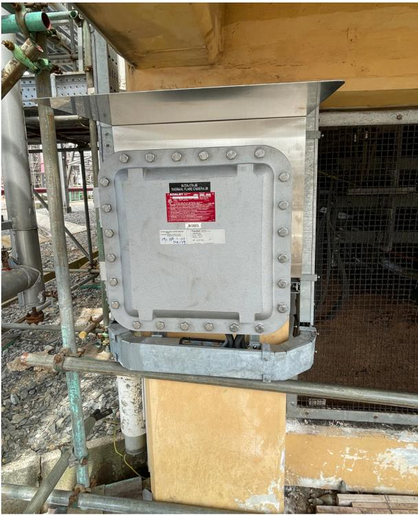
**Figure 3.** Field junction box used for power and fibre optic cable communications link.
