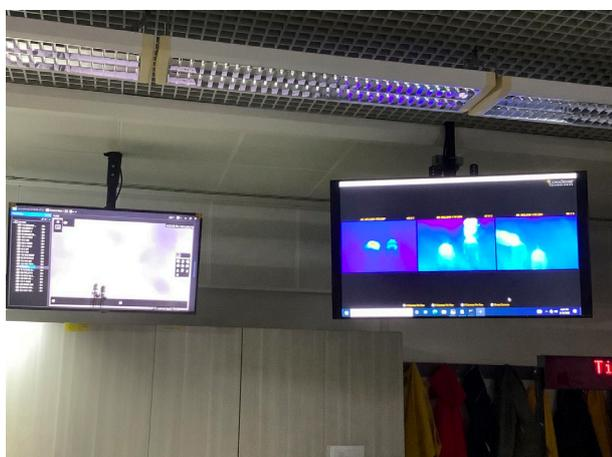
**Figure 2.** LCD panels showing IR flare monitoring in the plant control room.
