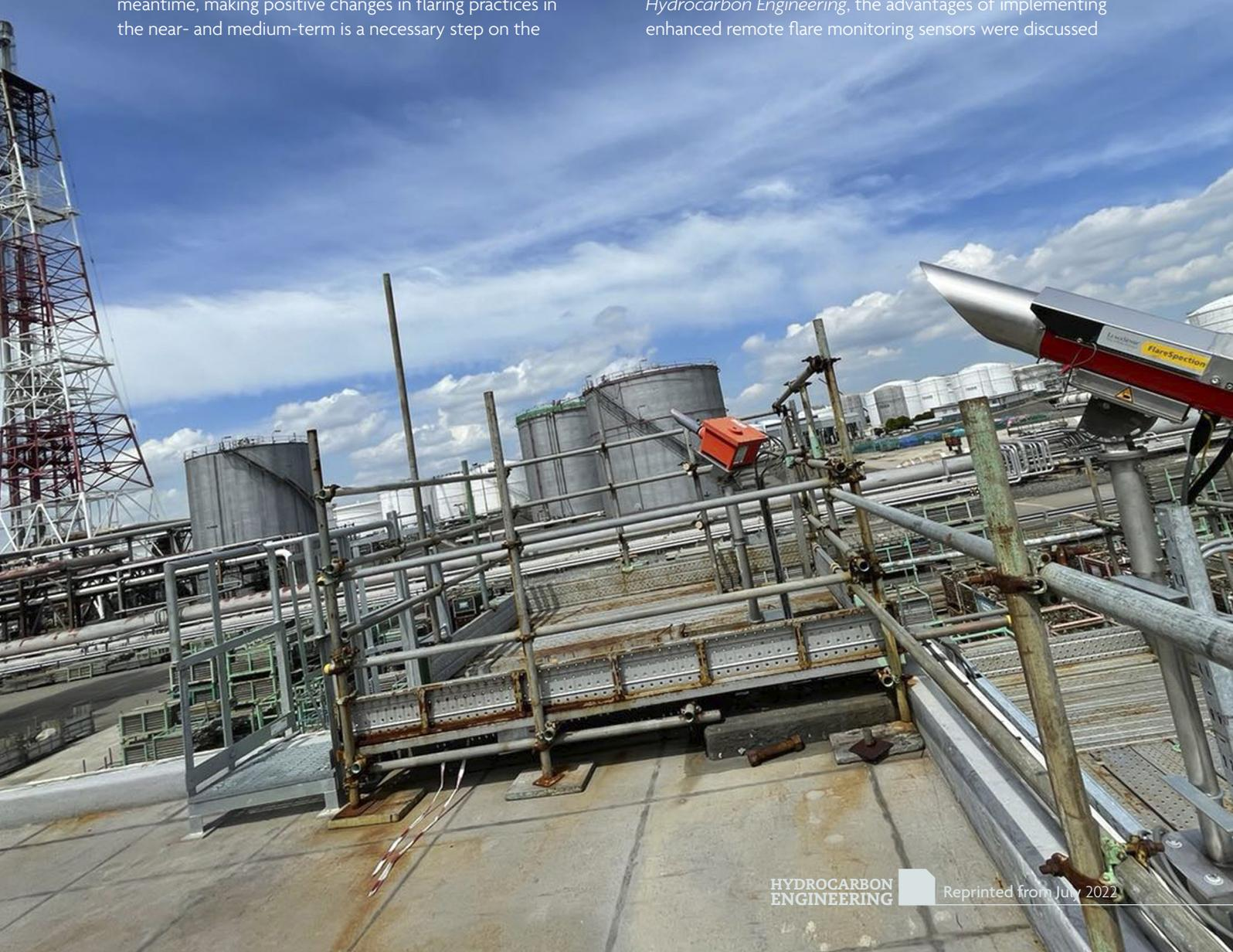
in the context of more effective flare monitoring functionality.<sup>1</sup> This article will instead consider an example of where remote flare monitoring using infrared (IR) cameras was implemented as a replacement for conventional thermocouple technologies.
