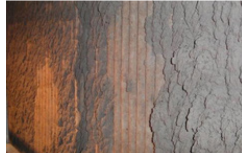
Figure 2: Slag on tubes
