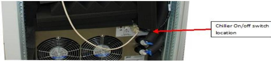
Figure 8: Chiller Power Switch
